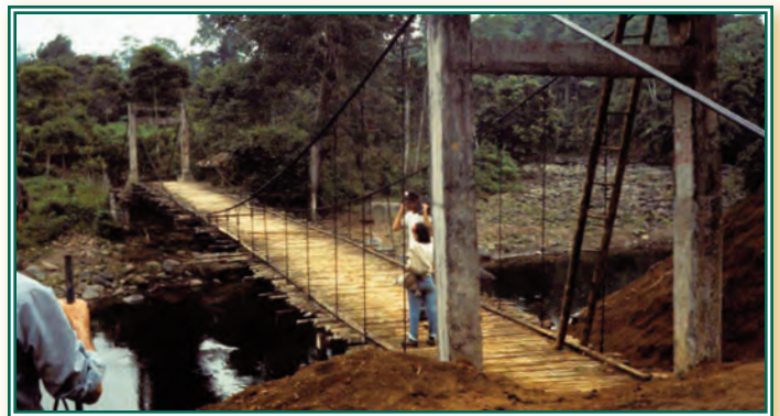
Peace Corps volunteers helped farmers build this bridge in Equador that could hold a loaded pickup.
